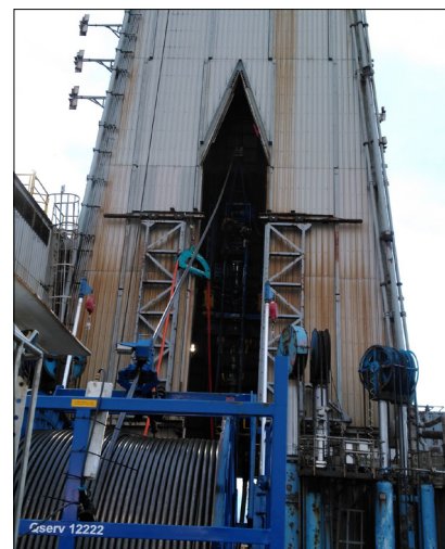
Coiled tubing rig up
